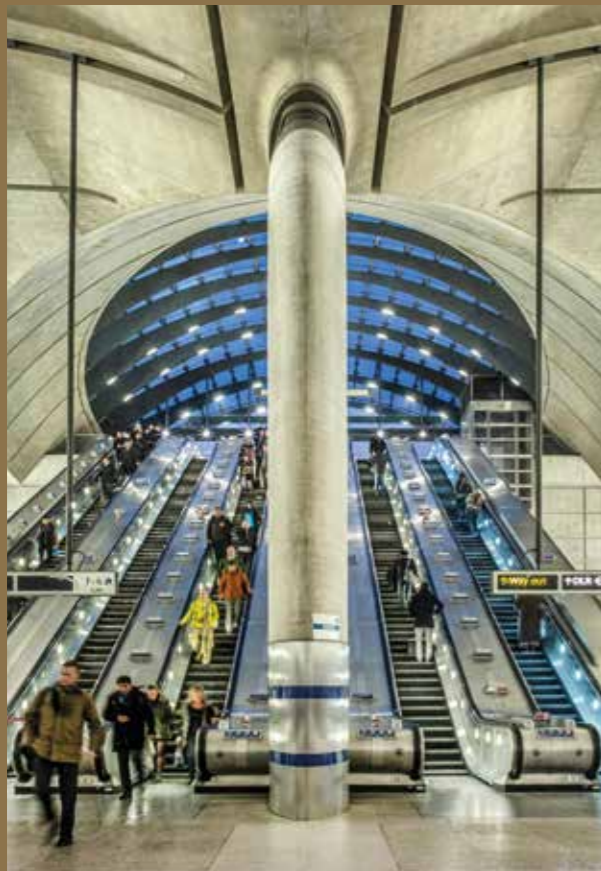
CANARY WHARF STATION
